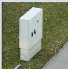
The new Sitraffic sX controller can be monitored and controlled via PC, smart-phone or tablet, including full remote maintenance functionality and convenient remote data upload. Following automated configuration (Plug&Play), the controller is directly included in the maps and lists of the Sitraffic smartGuard user interface.
